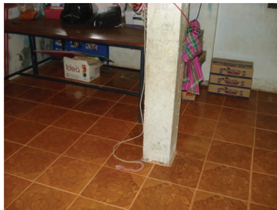
Pillar in the middle of the room
